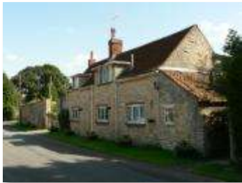
The late 18 th C Stone Cottage retains its character despite evolving to meet changing needs. Built originally as two cottages, it is now a single dwelling sporting a side extension, added or replacement chimneys, non-matching Victorian chimney pots, dormers and uPVC windows. Yet it still has tremendous charm and is perfectly integrated into the streetscape.
