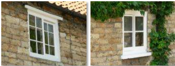
“Yorkshire sash” windows. Framing varies – the window on the left has no sill
